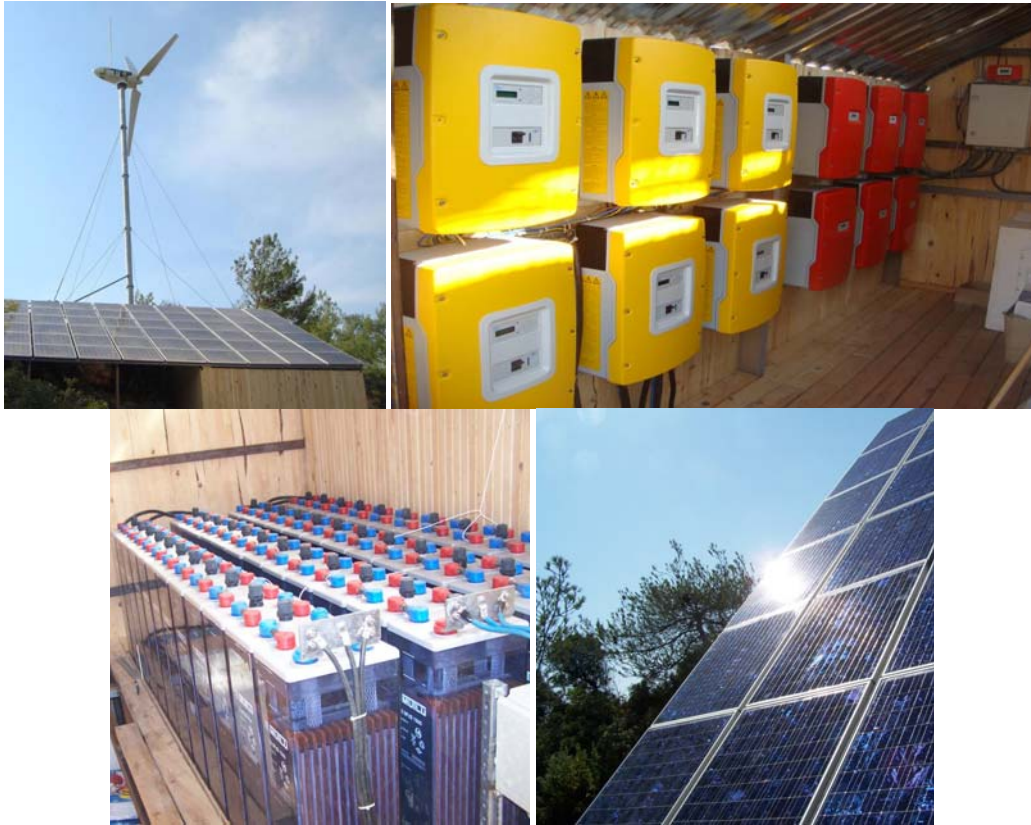
Fig.1. An off-grid PV hybrid system in Fethiye, Turkey.
